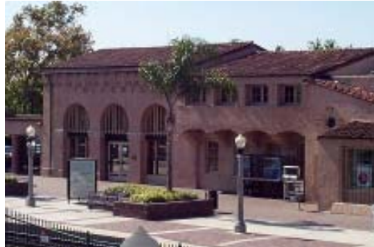
Transportation Center improvements, such as renovation of the historic Fullerton Depot, were redevelopment projects
